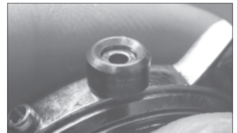
Figure 3. A bronze clock bushing was bored out to slip over the tube gasket.
