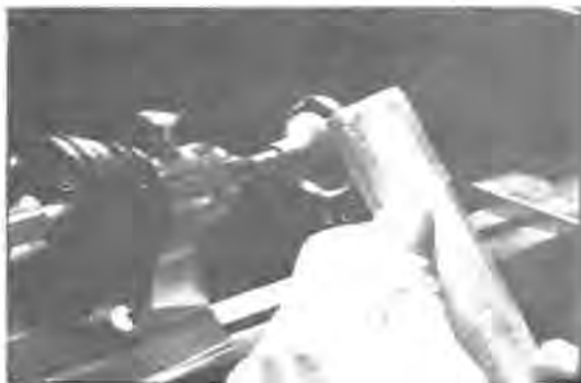
Figure 2. Dressing down a crystal with fine emery board.
