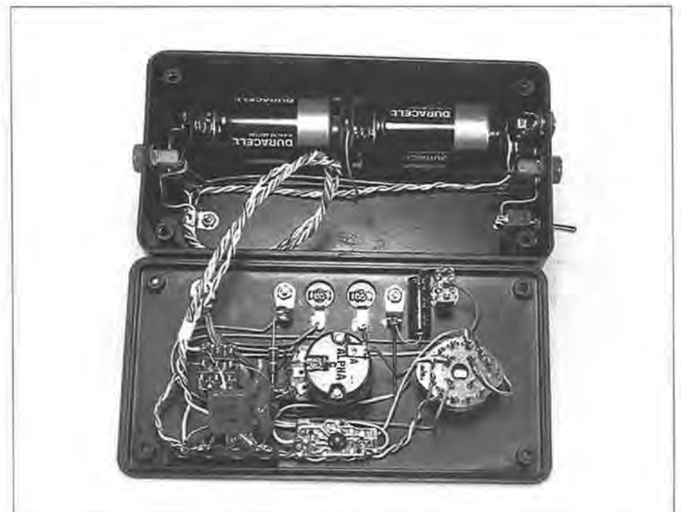
Figure 11. The test unit with all wiring completed and ready for use.
